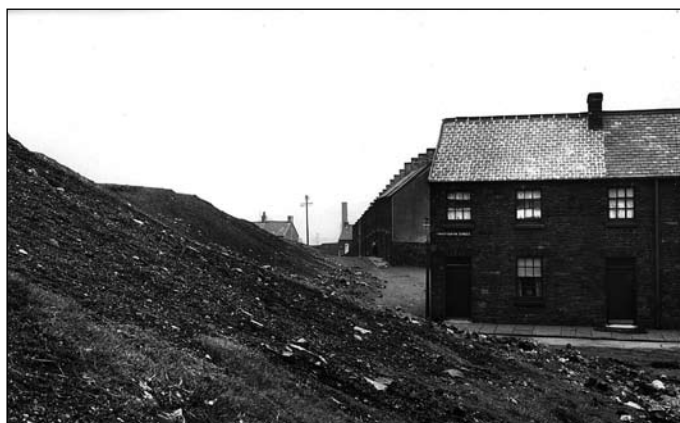
top Victoria Works, Dolgellau below Aberdyberthi Street, Swansea (West Glamorgan Archive Service)
