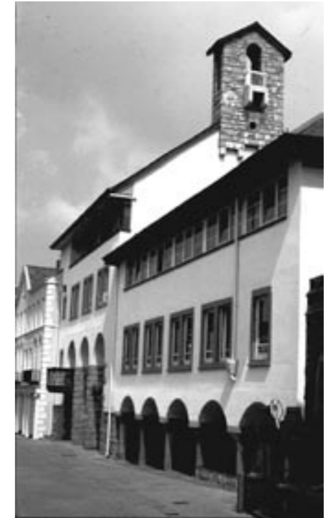
Fig 2 County Offices, Caernarfon A modern building using traditional construction in an historic context.
