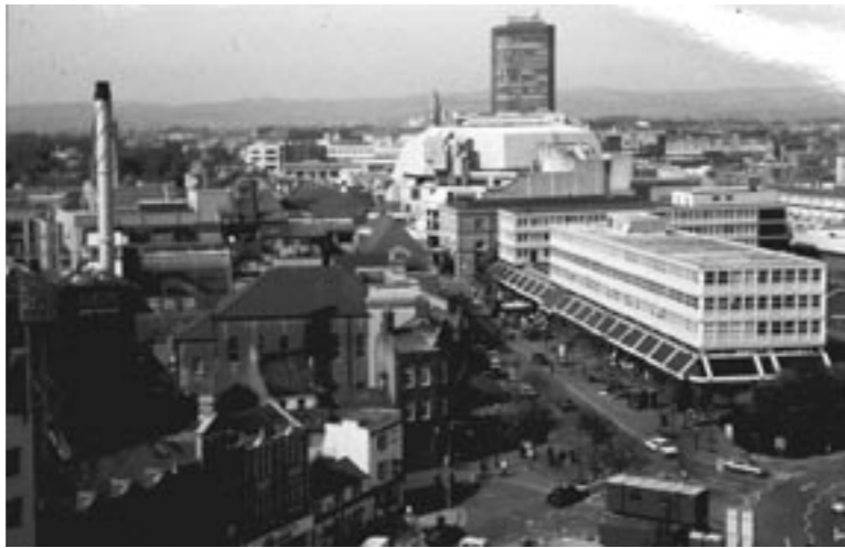
Fig 1 Cardiff: The Hayes Development and conservation pressures
