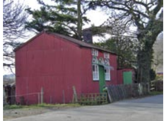
▲ Corrugated iron used as a building material Haearn rhyhog wedi ei ddefnyddio fel deunydd adeiladu
