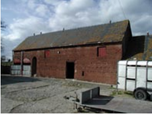
▲ Dolmelinau estate the red colouring comes from the crushed brick aggregate Ystad Dolmelinau daw'r llewyrch coch o'r gro o fri wedi'i falu
