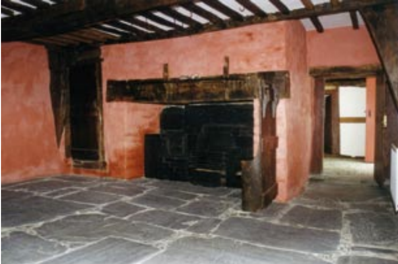
▲ Llanerch-y-cawr The 17th-century floor beams were strengthened and retained Cryfhawyd y trawstiau 17 ganrif a'u cadw (Mike Garner)
